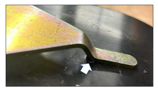
2.6 Using a  $\frac{1}{2}$  " drill, drill the hole made previously and tilt at 30°.
